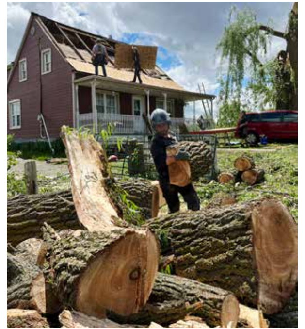
The roof of this old farmhouse in Très St. Rédempteur was ripped from the rafters, while trees around it were splintered.
